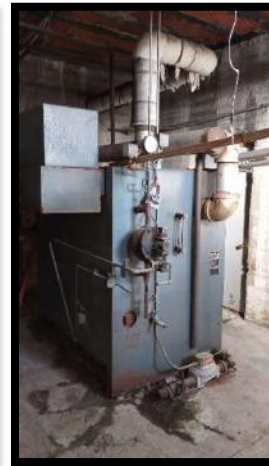
Picture 1: Obsolete boiler in west church basement space.
