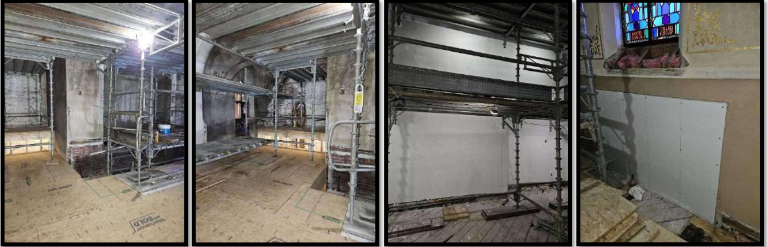
Picture 1: Choir loft Northwest Corner (West Stairs Removed)
