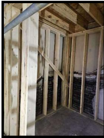
Framing the new bathroom space.
